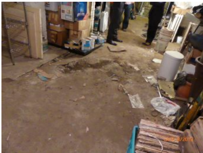
Dirt foundation floor
