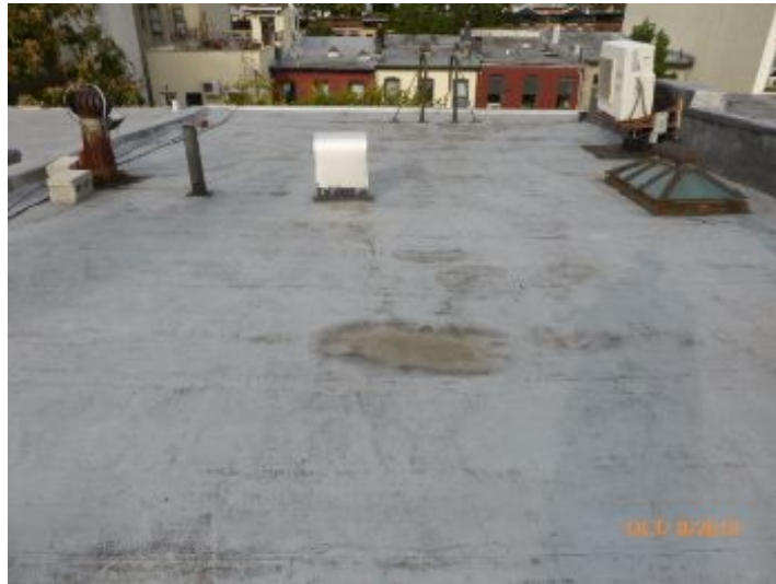
Roofing Roof Covering
