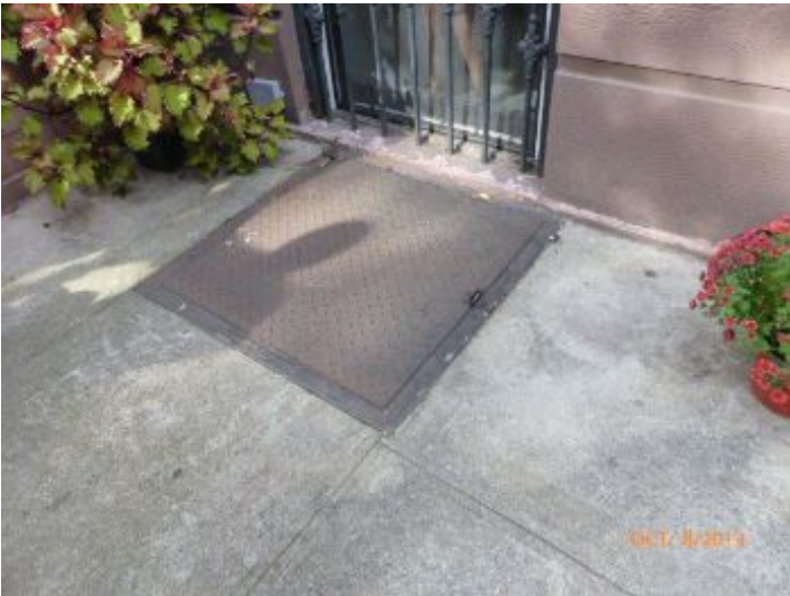
Ventilation shaft cover
