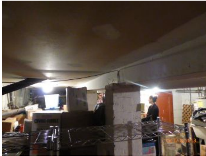
Full Ceiling installed in basement
